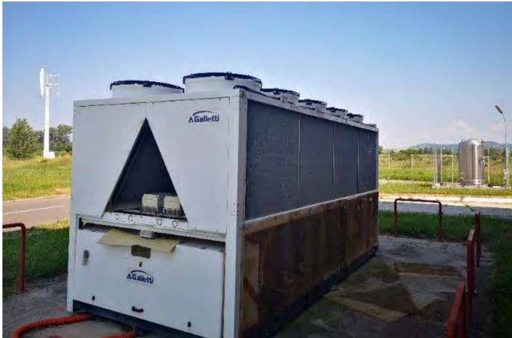
Figure 4.9 – Galletti Air-to-Water Heat Pump
