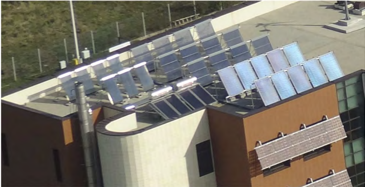
Figure 4.17 – ICSTM Solar Thermal Experimental Platform
