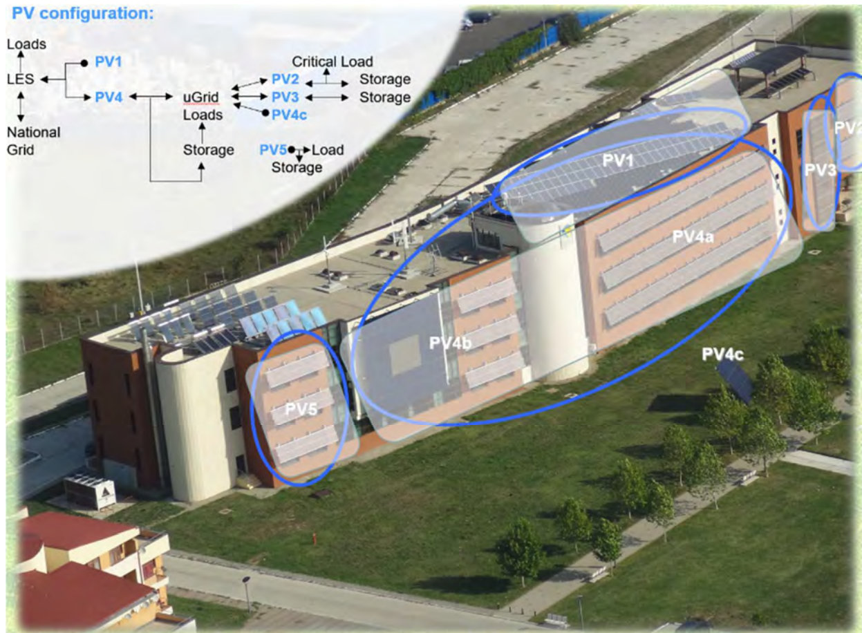
Figure 4.16 – Initial electrical configuration of the PV experimental platform
