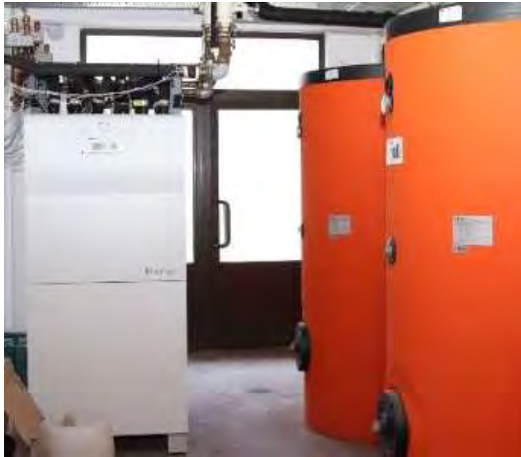
Figure 4.11 – Adsorption chiller coupled to a heat source
